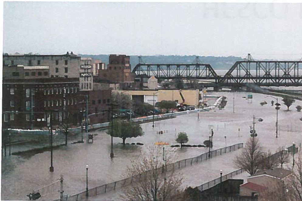
General Photo of HESCO Barrier Block Installation with Flood
