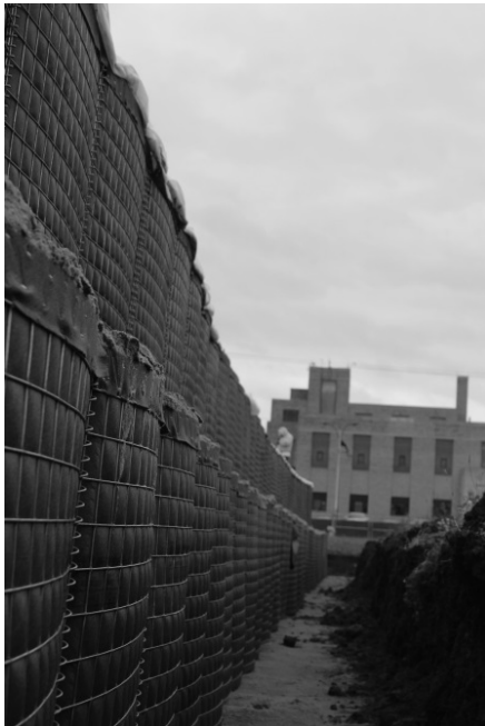
Figure 3-4 HESCO Barrier Blocks Used for Council Bluffs, IA Waterworks.
