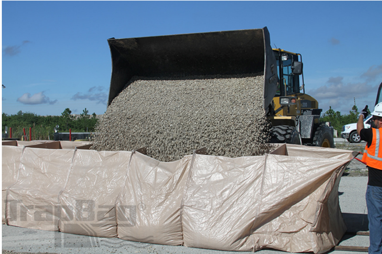
Figure 3-2 4-ft Tall TrapBag with Granular Fill
