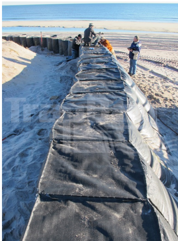
Figure 3-1 TrapBag with the UV Guards Installed
